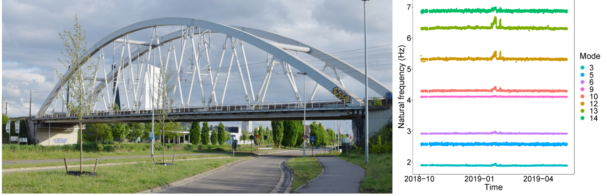
Figure 11. KW51 bridge from the north side (Anastasopoulos et al., 2022) and the considered natural frequency data.
