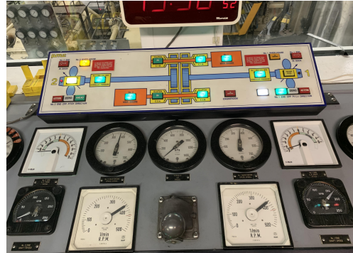
(b) Engine room
