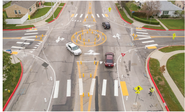
Temporary Roadway Enhancements such as paint and flexible posts/bollards are typically less expensive than concrete and may be installed to enhance traffic safety.
