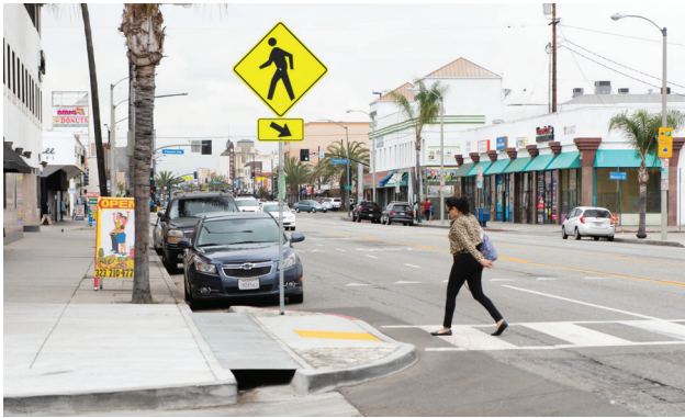
Curb Extensions (also known as bulb-outs) shorten the crossing distance for pedestrians, slow turning vehicles, and enhance the ability for pedestrians and motorists to see each other. Curb extensions can consist of paint and flexible posts or bollards and/or curb and gutter.
