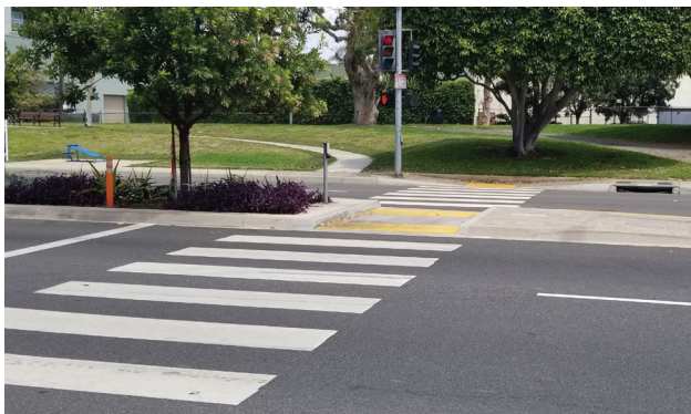
Refuge Islands provide a space within a median, mid-way through a crosswalk, for people to wait for a gap in traffic before continuing to cross a wide roadway.
