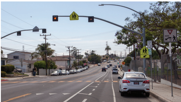
Pedestrian Activated Warning Beacons are flashing yellow lights that provide additional warning to drivers that a pedestrian is crossing the roadway.
