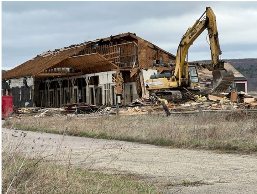
Environmental Hazard Remediation at Sacred Earth Parcel- Lab building demolition
