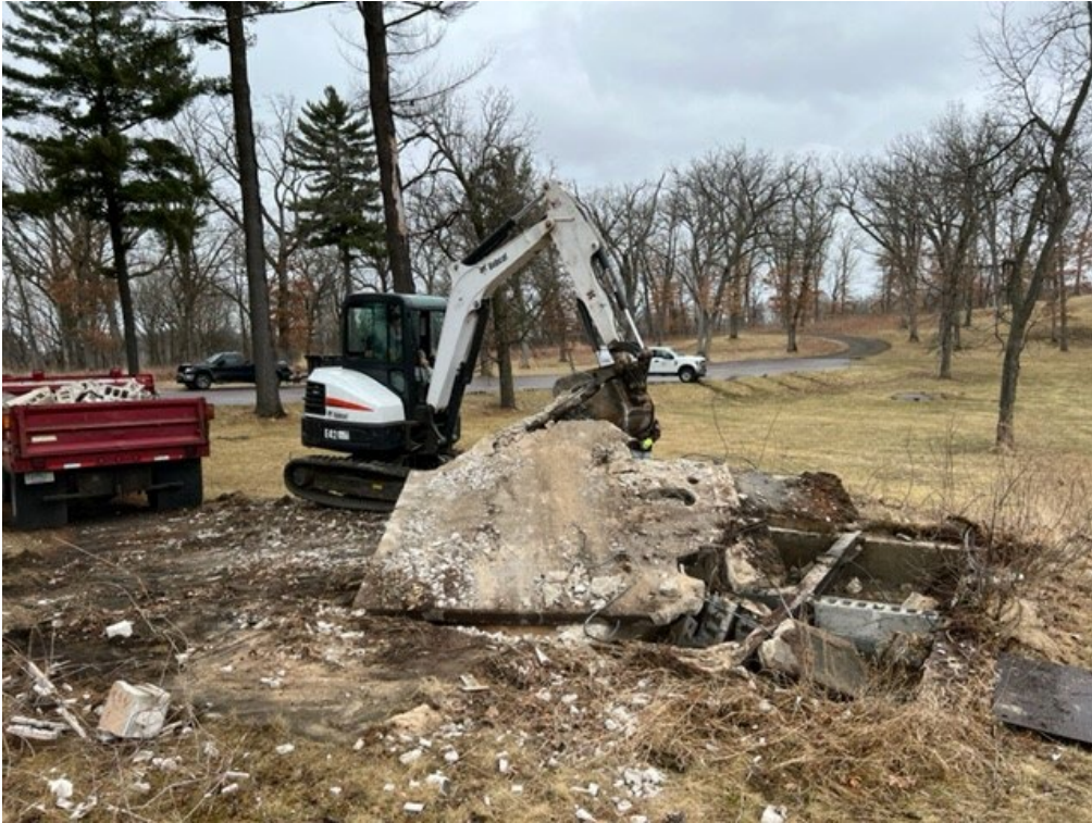
Environmental Hazard Remediation at Kingsley Bend Parcel- Pit toilet demolition
