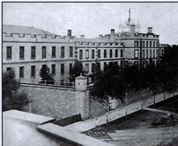
Auburn State Prison, homlokzat (Auburn, N.Y.)
