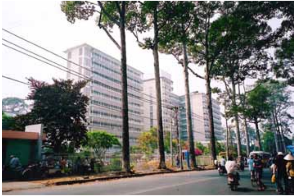
Figure 12: Chợ Rẫy Hospital, photograph by Huỳnh Vinh Thanh.
