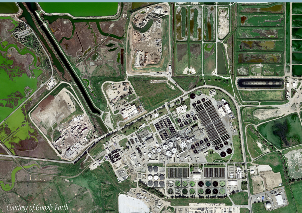
Photo to left: The San José-Santa Clara Regional Wastewater Facility, the largest facility in the Bay Area, is planning major improvements, including upgrades to treatment performance and flood management
