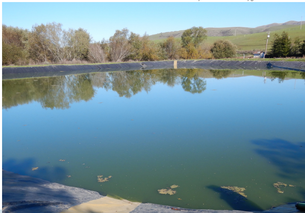
Photo below: Wastewater pond at Olema campground
