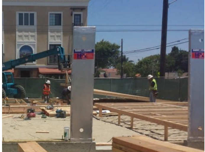
View of new construction at Café Camellia Site.
