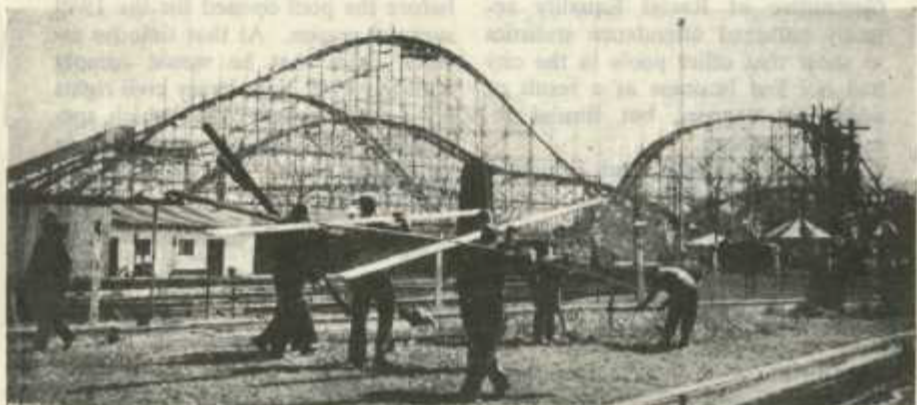
GENERAL VIEW of Palisades Park, New Jersey.
