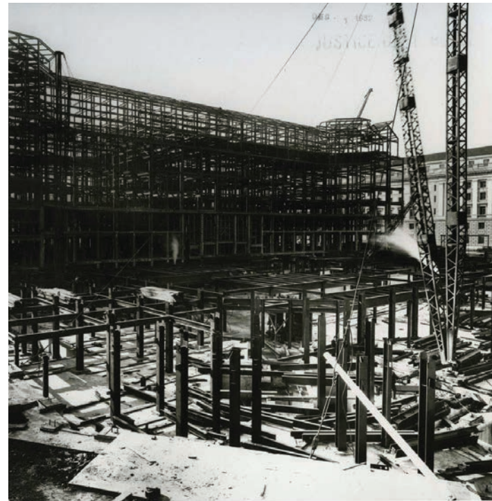
Looking southwest at the steel frame of the Department of Justice Building, December 1, 1932. The 10th Street side of the IRS building can be seen on the right. 27
