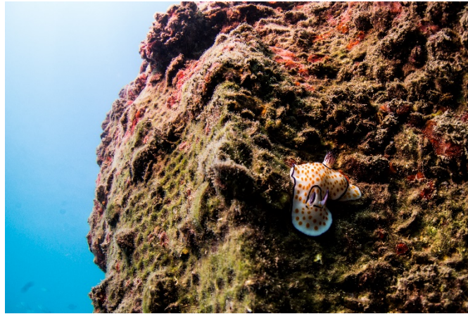
Figure 21: Example of marine growth on an EConcrete armor unit in Haifa Israel. Source: https://econcretetech.com/econcrete-solution/
