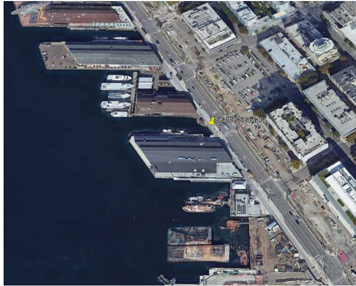
Figure 13: Seattle Seawall site. Source: Google Earth
