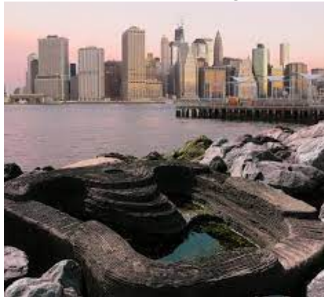
Figure 12: ECOconcrete tidepool units. Source: https://econcretetech.com/projects/brooklyn-public-park-renovation/
