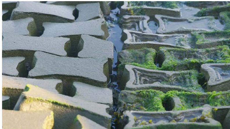
Figure 22: Effect of using enhanced concrete and surface texture to enhance habitat. Source: https://econcretetech.com/blogcat/ecological-concrete-block-mattresses-acbm-scientific-study/
