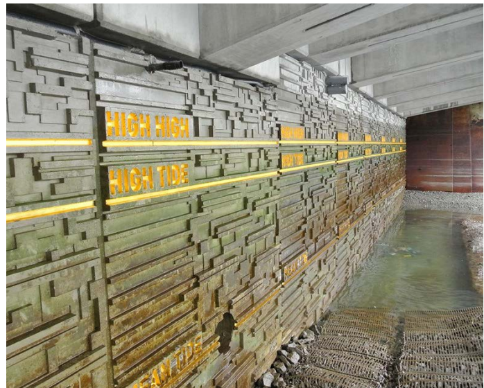
Figure 20: Example of surface roughness used in the Seattle Seawall project. Source: https://waterfrontseattle.org/waterfront-projects/seawall
