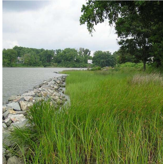
Figure 19: Example marsh sill http://ccrm.vims.edu/livingshorelines/design_options/structural.html
