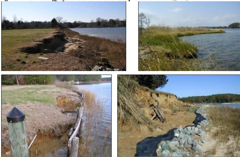
Figure 4: Low-energy systems and failed shore protection structures
