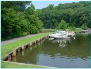
Pre-construction site with bulkhead and minimal aquatic habitat. Photo: Rich Takacs, NOAA Restoration Center
