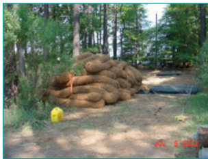
Natural fiber logs, pre-installation. Photo credit: Rich Takacs, NOAA Restoration Center
