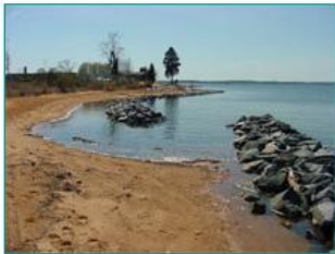
Post-construction segmented rock sill. Photo: Rich Takacs, NOAA Restoration Center
