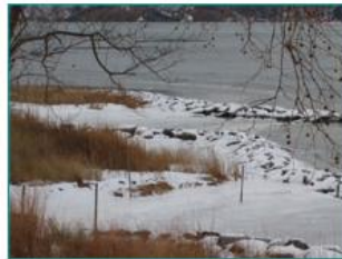
Low-crested segmented rock sill with marsh grasses. Photo: Alison Ward-Maksym, NOAA Restoration Center
