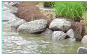
Natural fiber log held in place by a rock footer. Photo: Chesapeake Bay Foundation
