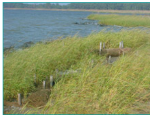
Natural fiber logs, post-installation. Photo credit: Rich Takacs, NOAA Restoration Center
