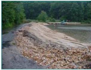
Bulkhead removal, shoreline regrading, and filling process. Photo: Rich Takacs, NOAA Restoration Center
