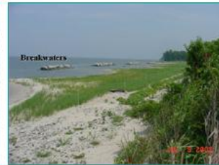
Offshore segmented living breakwaters. Photo: Rich Takacs, NOAA Restoration Center
