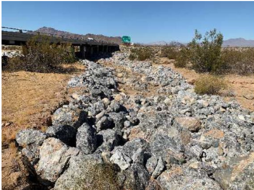
Photo 2 Area north of the westbound lanes of I-40 looking west.
