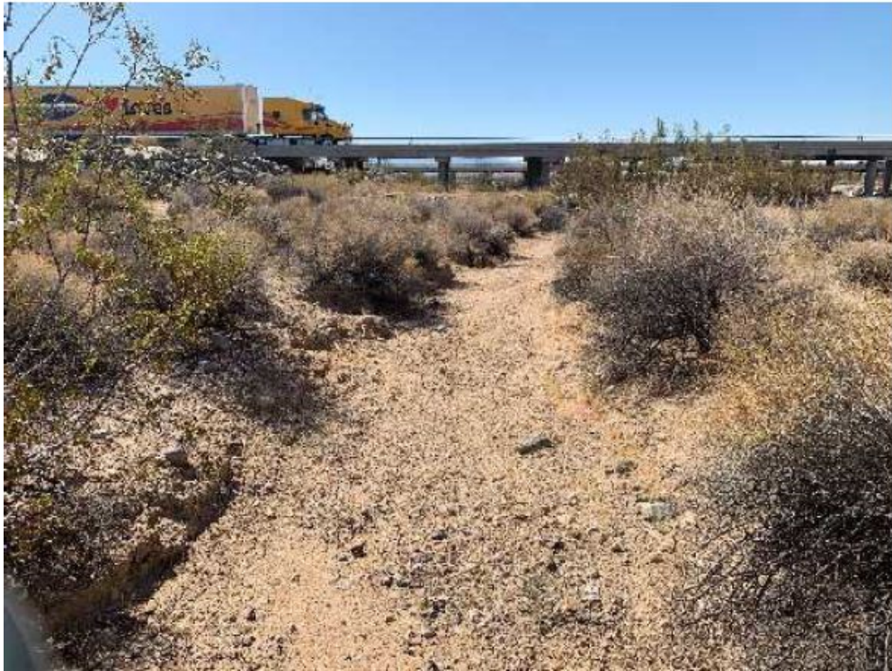
Photo 1 East levee north of I-40 looking downstream (south).
