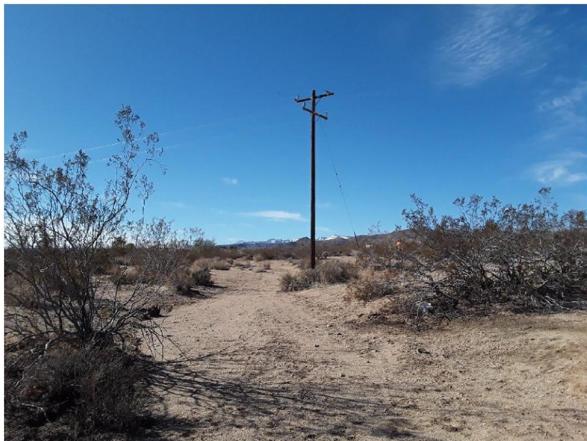
Figure 4: Pole overview. Photo facing southwest (upstream).
