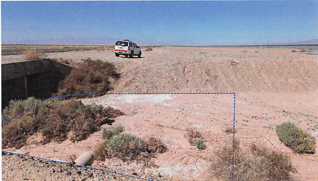
Photo F1. Imperial County, SR 111, PM 50.65 at Frink Wash. Proposed staging area upstream of the roadway, view northwest towards the west bank.
