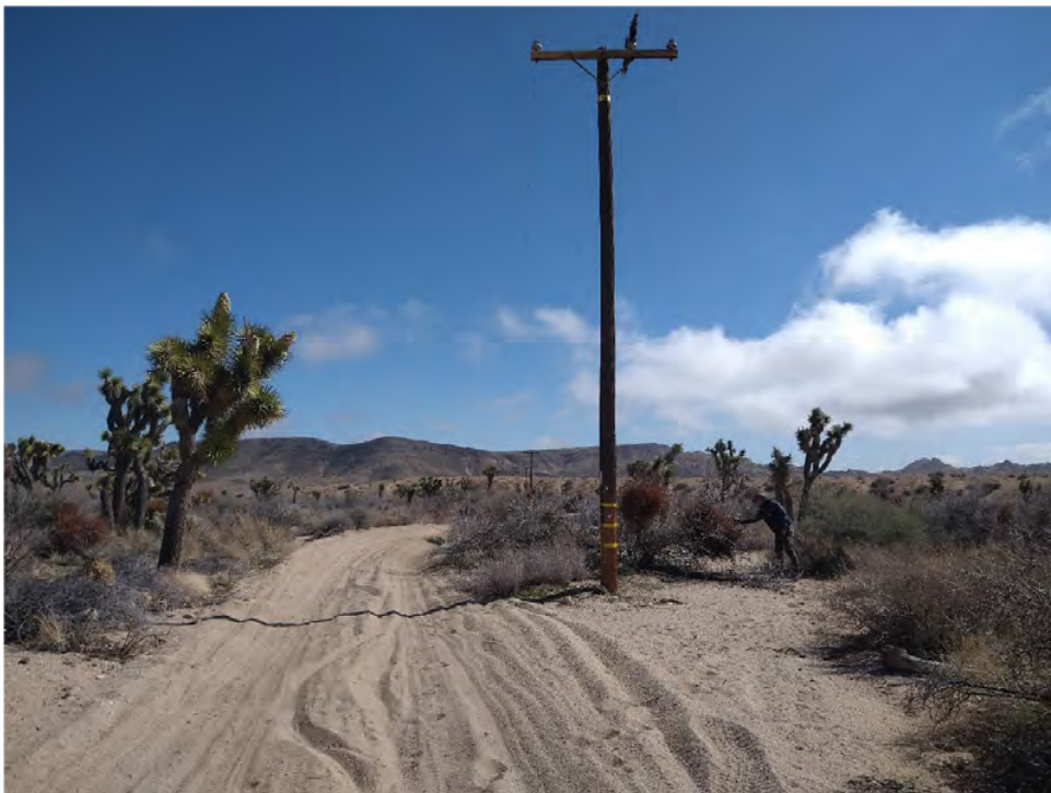
Photo 2. Pole 2009916E, Overview Facing East
